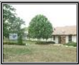
Smarr Hall (Building 291)
