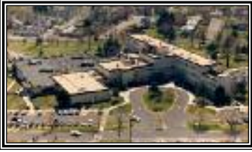
Patterson Army Health Clinic (Building 1075)
