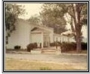
Blair Hall (Building 259)
