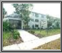
Black Hall (Building 360)
