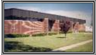
Van Deusen Library (Building 502)
