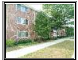
Moorman Hall (Building 362)
