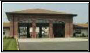
Fire Station (Building 2560)
