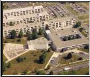
Pruden Auditorium and Mallette Hall
